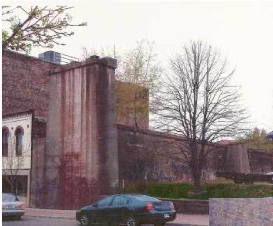
Removal of the concrete abutment looking West
