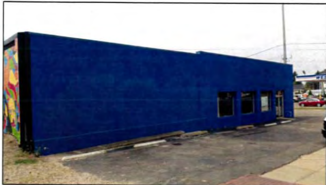
Vacant Commercial Building
