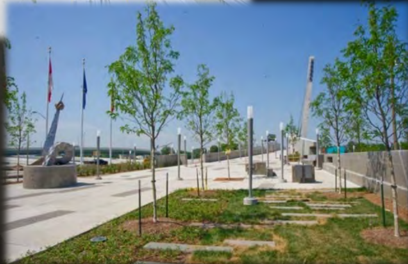
Bagley Street Pedestrian Bridge over I-75 Gateway Project, Detroit , Michigan
